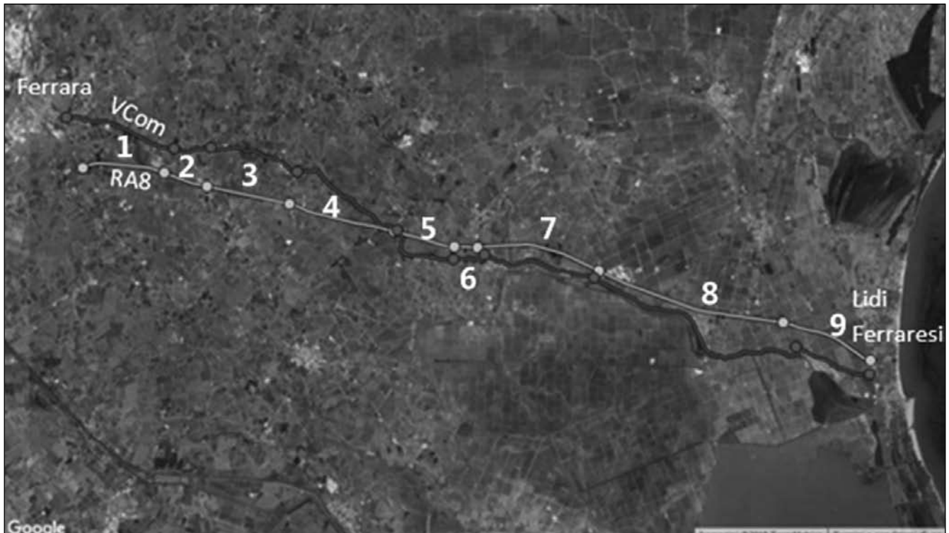
Fig. 2. Satellite image of the study area with details of the subdivision into 9 sections of the two roads Via Comacchio (VCom) and RA8. Scale 1: 300.000, Google images processed with QGIS 2.14.22 Essen.
